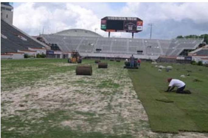
Figure 2. Laying sod over existing sprigs on June 21, 2006.
